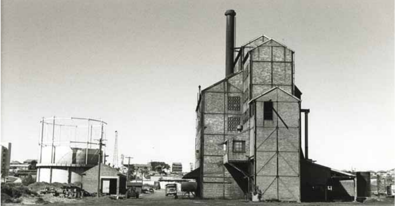
The Wollongong Gas Works in Charlotte Street dominated the area and was ugly. Today, most of the land is owned by The Collegians Club.
