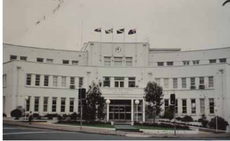
The Wollongong City Council Chambers about 1950s
