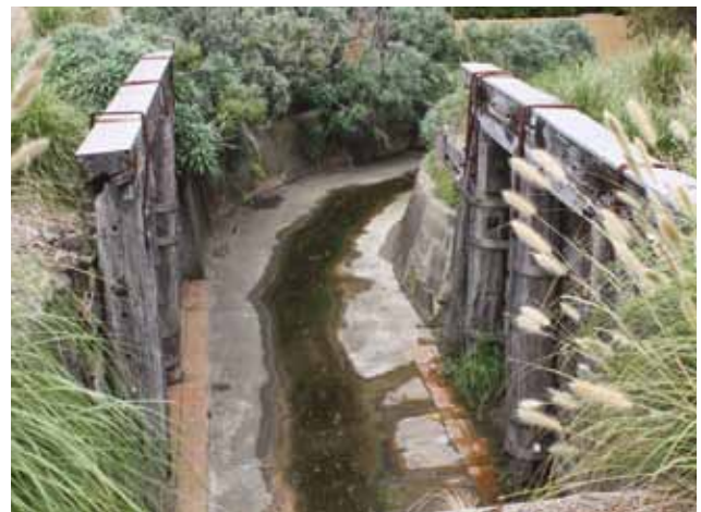
A section of the Mount Keira Tramway that has been preserved at Osborne Park, Wollongong
