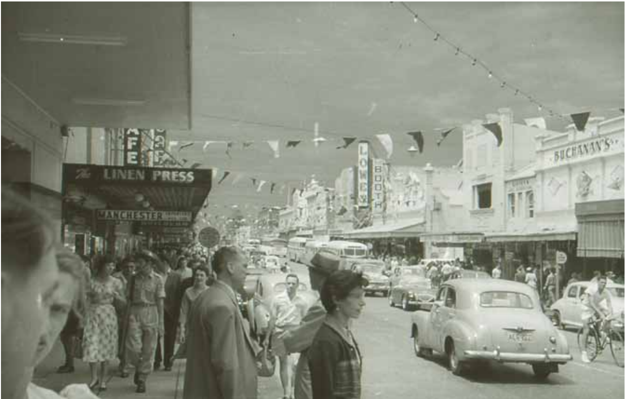
Wollongong's famous Crown Street in the late 1950s. Population growth and an influx of migrant hostels led to a high demand for builders to construct homes
